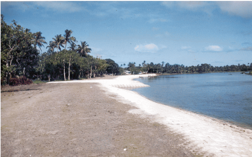
Figure 1: Rewa River Bank Protection
