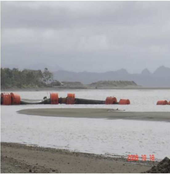
Navua river mouth dredging
