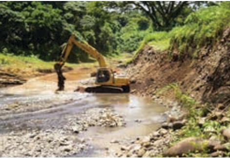
Gravel and river rock extraction © Dick Watling.
